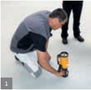
1 Evaluate and test the subfloor
