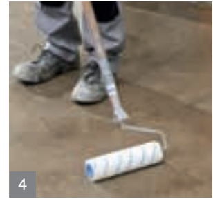
4 Apply a primer/scratch coat
