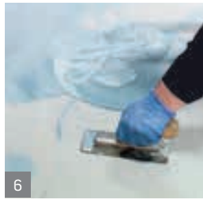
6 Apply the self-smoothing floor
