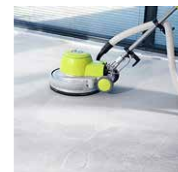
Grinding of the substrate and subsequent vacuuming
