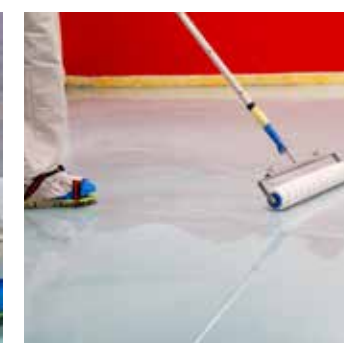
In the last step the second sealing coat is applied
