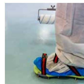
Applying the first sealing coat with a nylon roller
