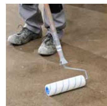
Primer is applied
