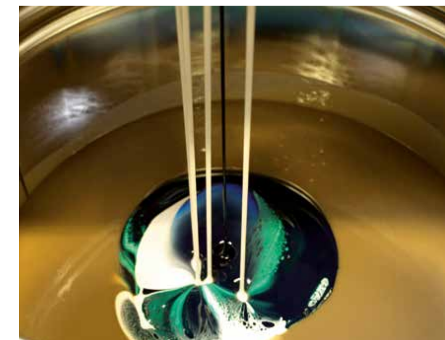
Mixing the self-smoothing floor components
