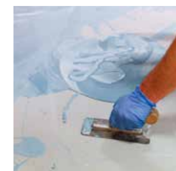
The self-smoothing floor is applied with a trowel
