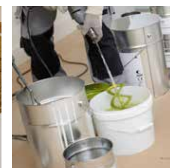
Mixing the self-smoothing floor components
